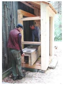
In the first picture, Mark is driving an oak peg into a beam to secure it to the vertical corner post. Note the granite curb stones beneath the sill. The one on the right shows Mark and me moving the "box" into the nearly completed privy.
